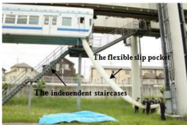
Fig. 1 The independent staircases and flexible slip pocket of Chiba Urban Monorail in Japan
